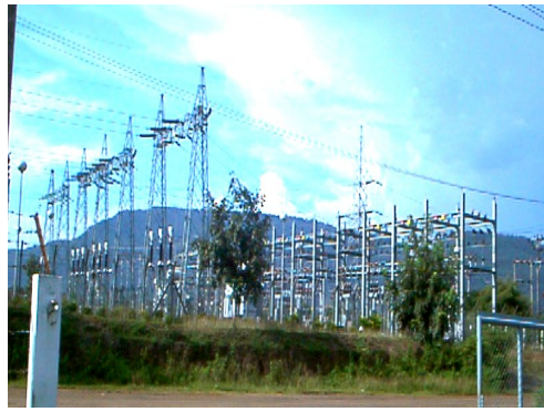
Substantial potentials for energy generation existing
